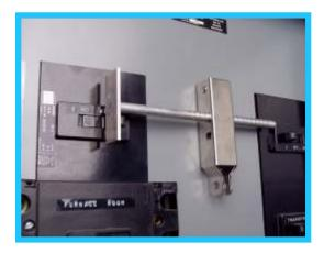
• Some large frame breakers may require a Large Breaker Lockout Set. Generally, the Large Breaker Lockout is appropriate when the standard rail assembly pins are not long enough to engage the breaker handle. In this case, the circuit could not be turned off for the photo and so the pin is positioned to hold the breaker on. The position of the lockout device between breaker columns enables it to lockout the circuit to the right or to the left.
