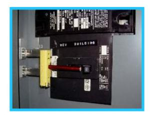
• Sometimes, due to panel configuration, a rail assembly cannot be mounted directly onto the deadfront panel. In these situations, "L" shaped Offset Brackets can often be used to install the rail assembly. The Offset Brackets mount with self-tapping screws onto a panel surface perpendicular to the deadfront, and extend out to provide a base for installation of the rail assembly. In this image, a short rail is mounted on Offset Brackets to engage a large frame breaker handle.
