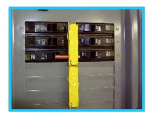
• Standard two-column panel with the rail installed in the center. One-Way Pins are used to lock out one circuit, Two-Way Pins are used to lockout opposing circuits. It is a good practice to install Circuit-Safety for the capacity of the panel rather than the currently used circuits.
