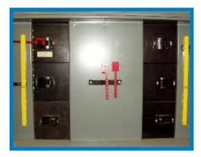
• Depending on the spacing between columns and the panel space available for a center mounted rail assembly, some panels require the installation of two Circuit-Safety rails (one for each column). In this case, the center of the panel is raised, requiring rail assemblies to be mounted to the "outside" of the breakers.
